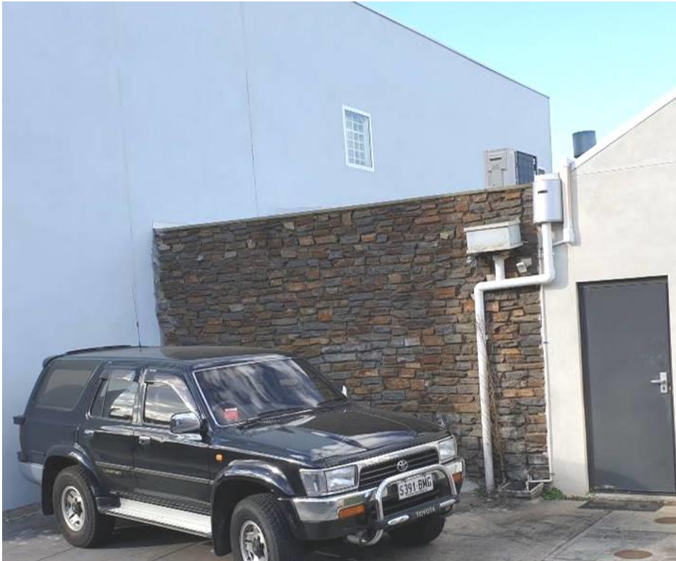
Photo 9.4.1 – Window located adjacent eastern boundary
