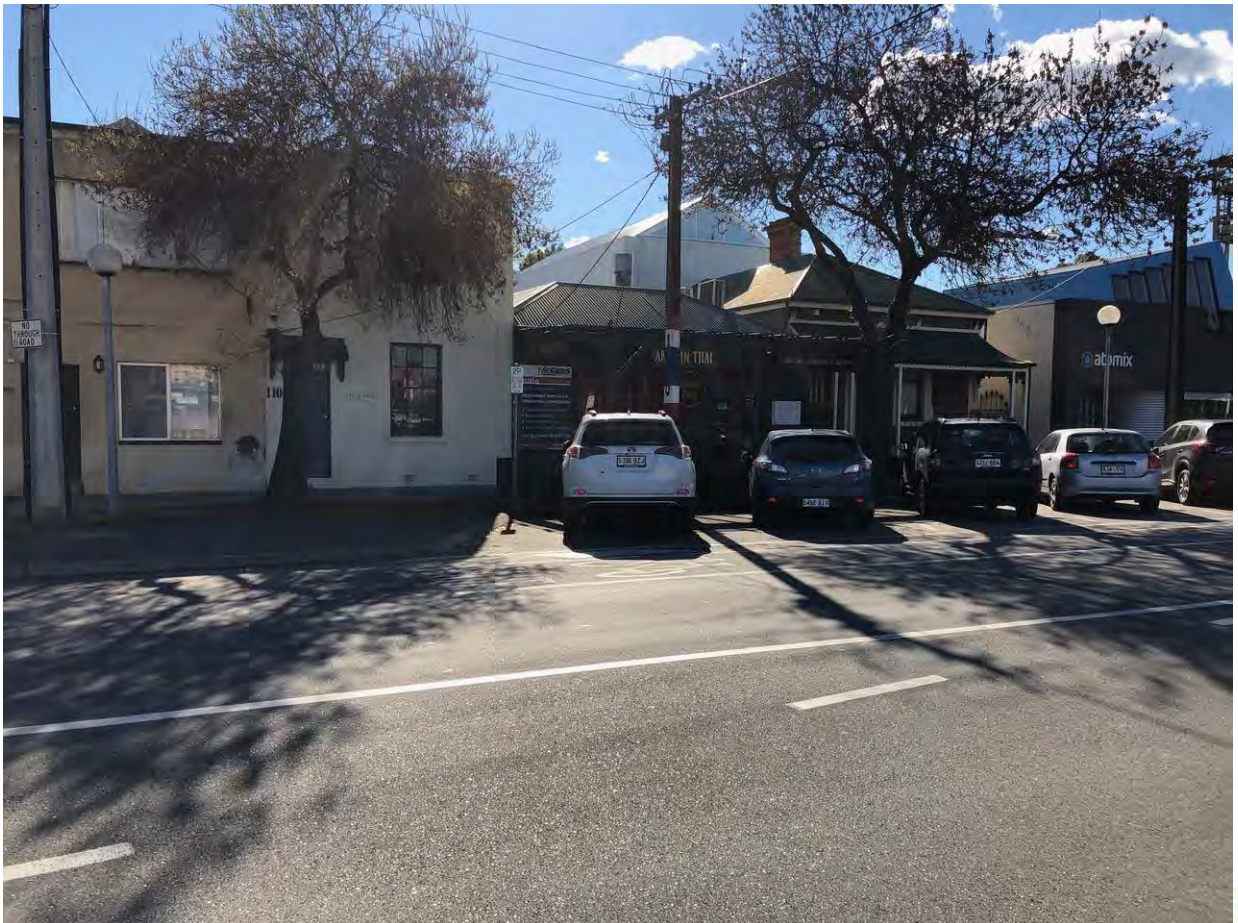
Figure 1: View of the subject land and the adjoining buildings to the east and west
