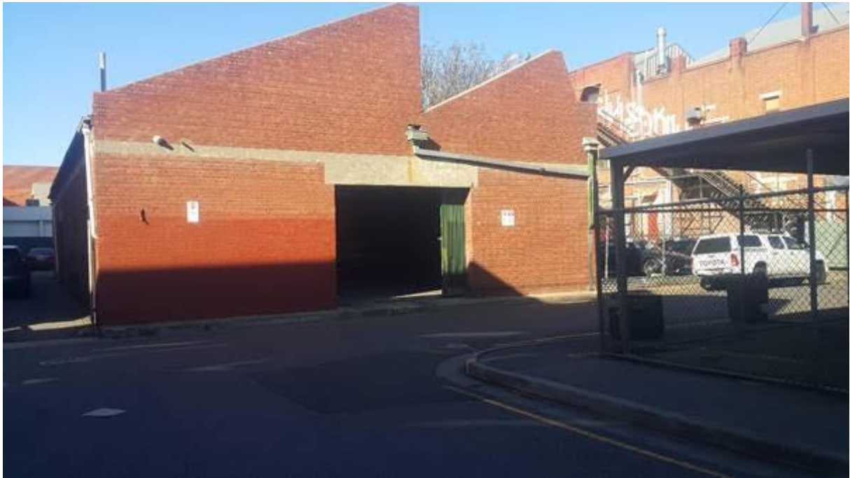
Photo 1 – Existing warehouse building on subject site, looking east
