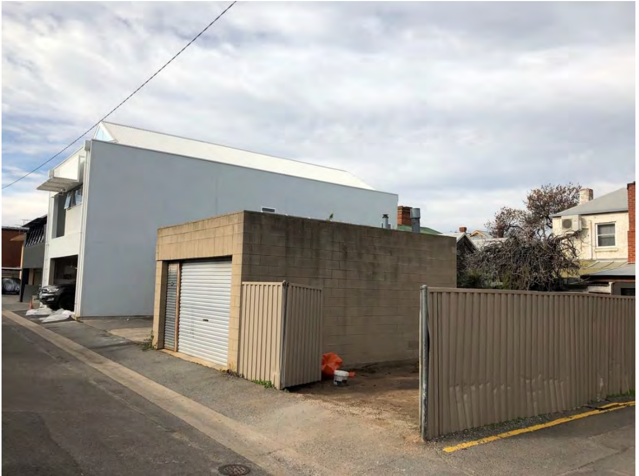
Figure 3: Existing two storey boundary wall at 104 Tynte Street North Adelaide
