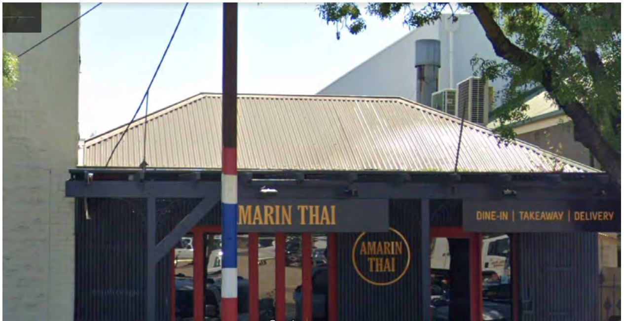
Figure 5: Existing flue location on eastern boudnary
